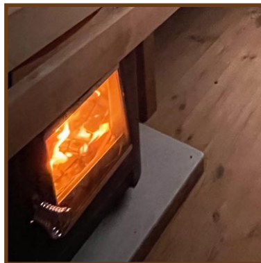
Once the fire is well started, you can add 3 logs. • 20 minutes later, you will put 3 logs
