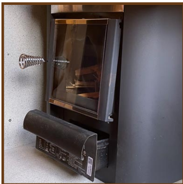
Open the ash pan slightly to increase the draught during lighting. Close it again when the sauna reaches 60°.
